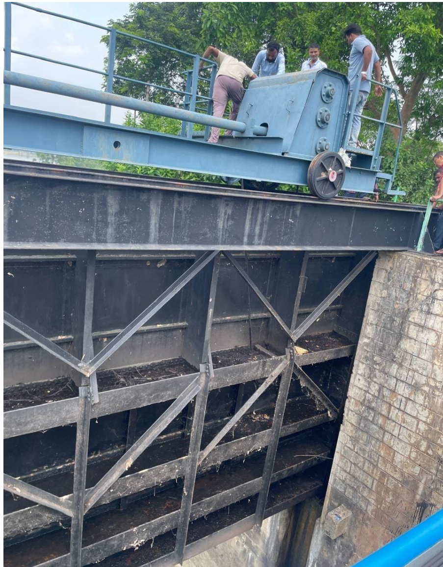
Existing manual trally and stoplog gate of spillway
